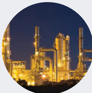
Energy and Industrial
