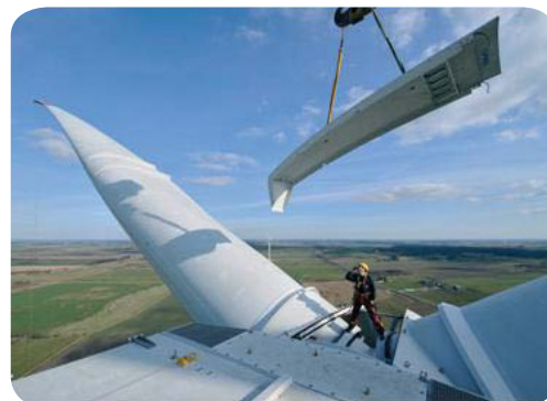
Bachmann's electric wind turbine control system is housed adjacent to the main turbine, pictured here during installation.
